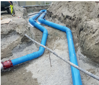
OPVC pipes and fittings installation
