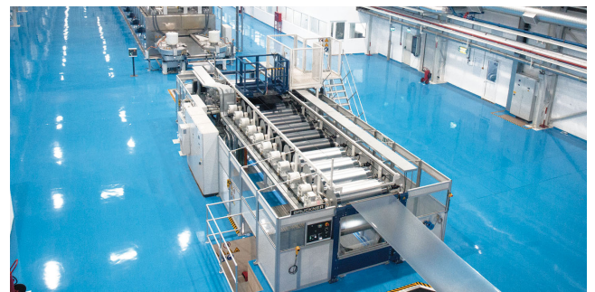
One of the reasons for Polibak's decision to team up with Brückner again: Perfectly working 8.7m BOPP line in İzmir
